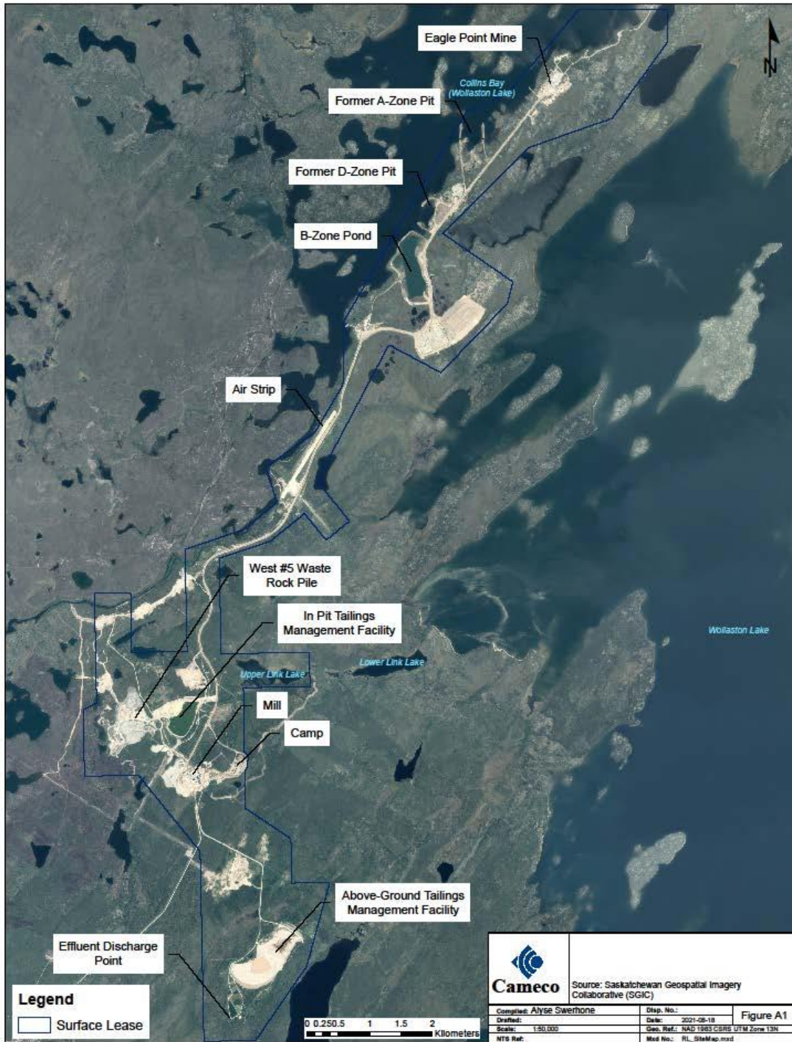
Figure 1.3: Aerial view of the Rabbit Lake Operation [24]
