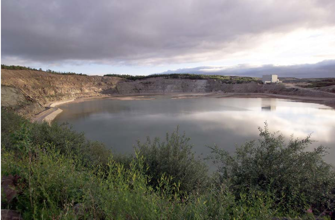
Figure 1.1-5: Rabbit Lake In-Pit Tailings Management Facility (RLITMF).
