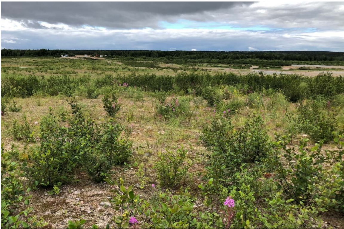
Figure 1.1-4: Rabbit Lake Above Ground Tailings Management Facility.
