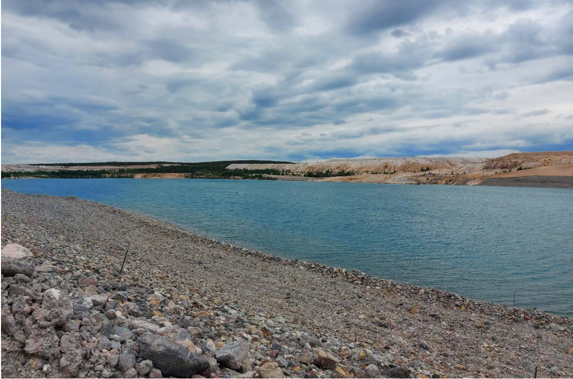
Figure 1.1-2: Key Lake Deilmann Tailings Management Facility.
