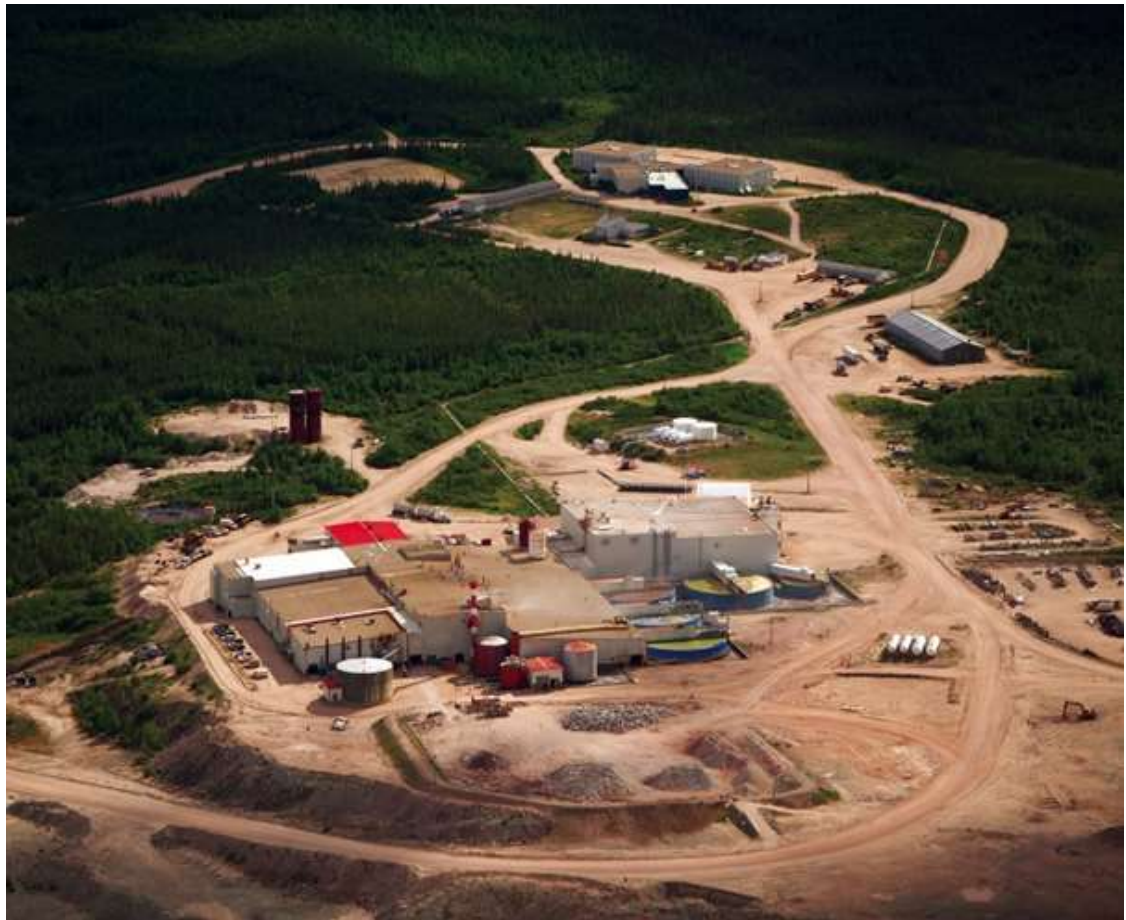
Figure 5.1: Rabbit Lake Operation - aerial view of mill
