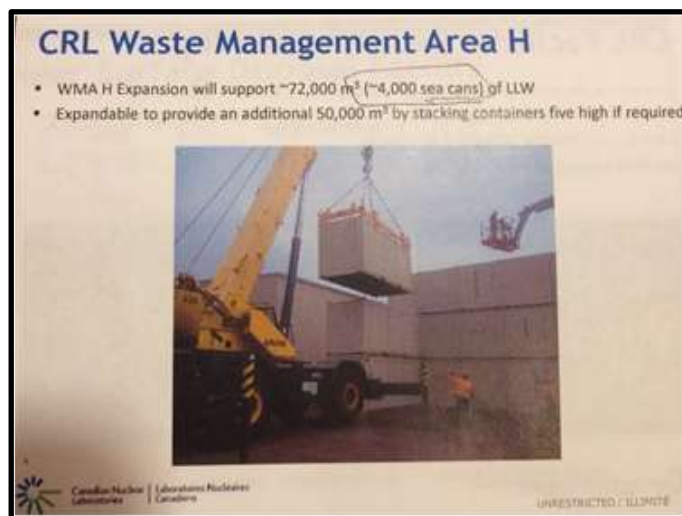
Figure 3: Waste Containers Destined for Disposal in the Mound
