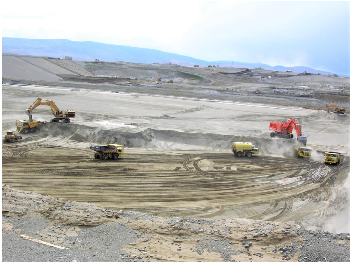
Environmental Restoration Disposal Facility – Super Cells 9 & 10 Construction
