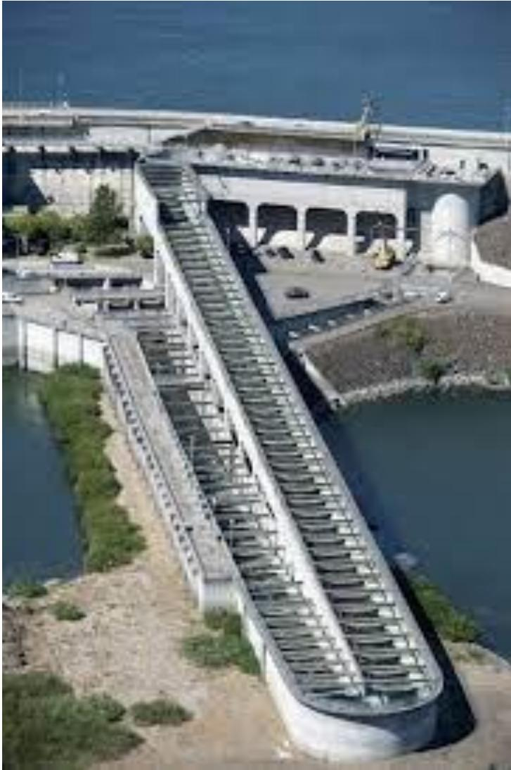
**Figure 6.** Dalles Dam East fishway used by White Sturgeon on the Columbia River.
