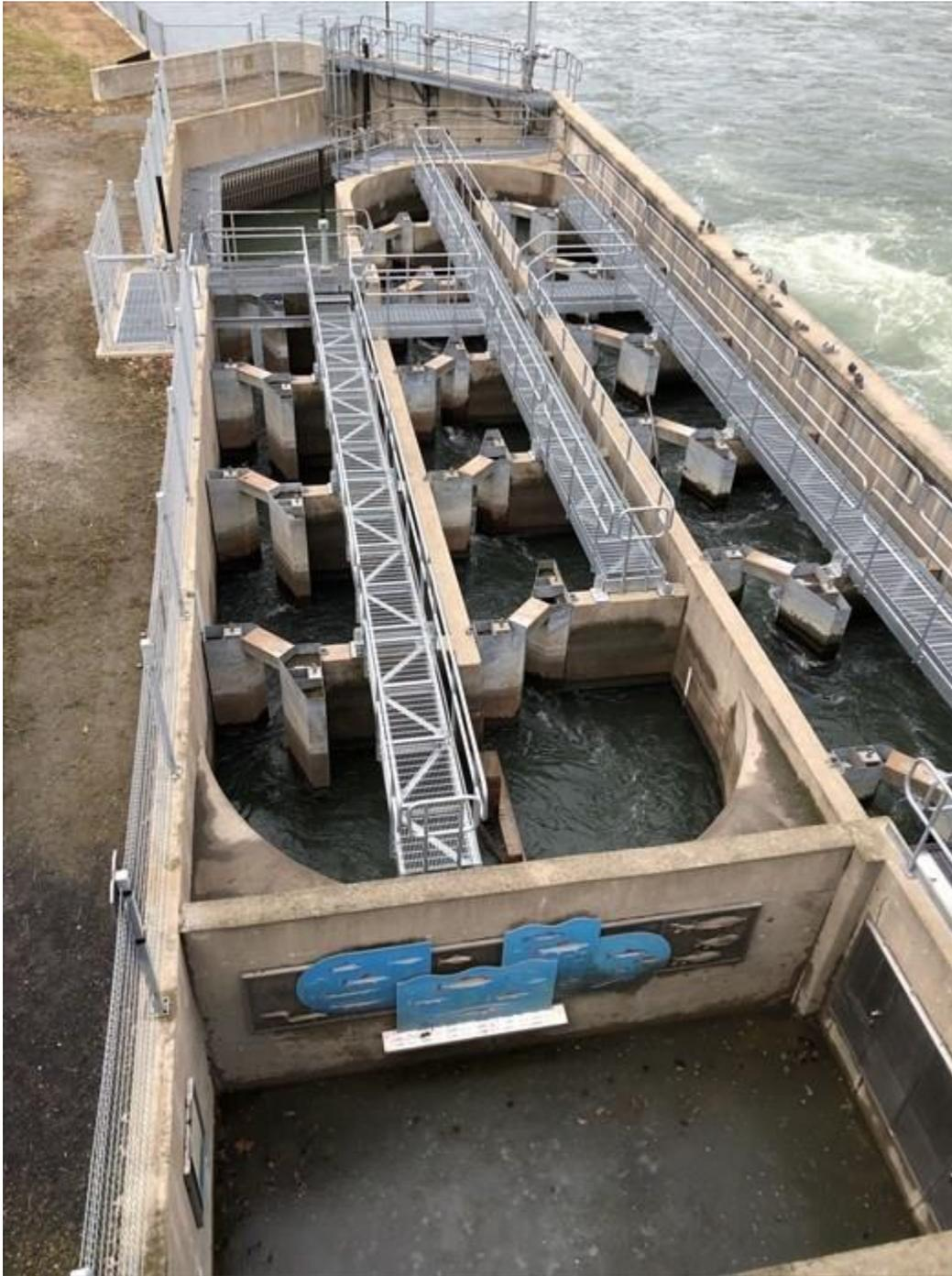
**Figure 4.** Vianney - Legendre Fishway at St. Ours Dam on the Richelieu River in Quebec. A vertical slot fishway design.
