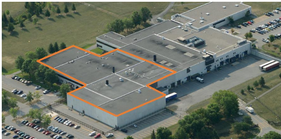
Figure 1: Aerial view of Nordion’s Cobalt Operations Facility (outlined in orange) (Source: Nordion (Canada) Inc.)
