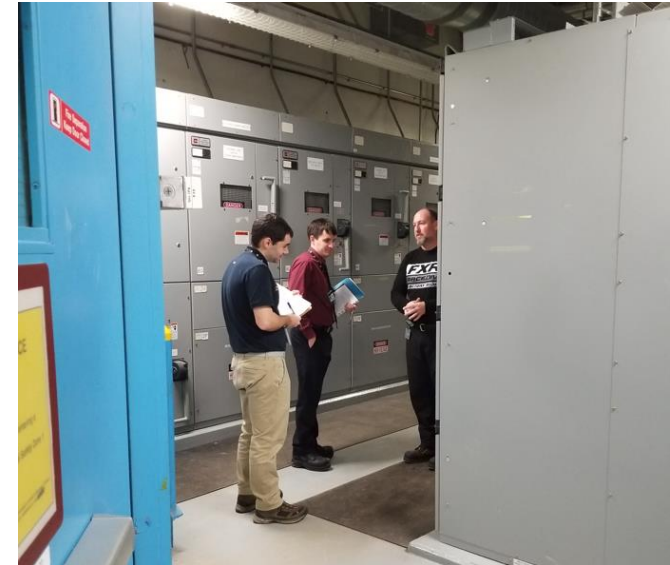
CNSC staff performing an inspection at Chalk River Laboratories (CRL)
