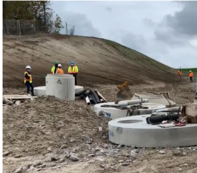
CNSC staff performing an inspection at Port Granby Project (PGP)
