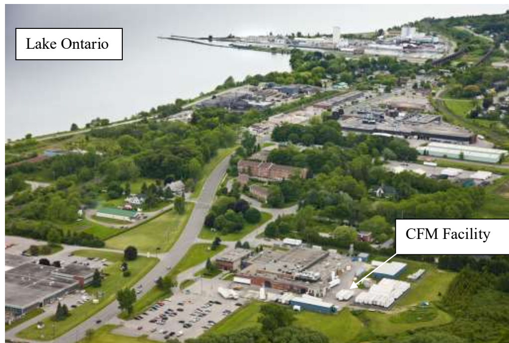
Figure 1 – Aerial view of the CFM facility, located in Port Hope, Ontario
