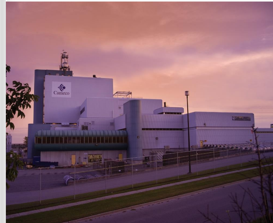
Side view of Port Hope Conversion Facility Source: Cameco
