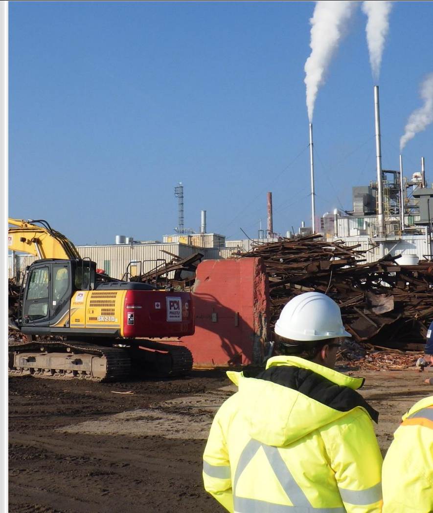
CNSC inspector observing demolition activities at Centre Pier in Port Hope, 2019.
