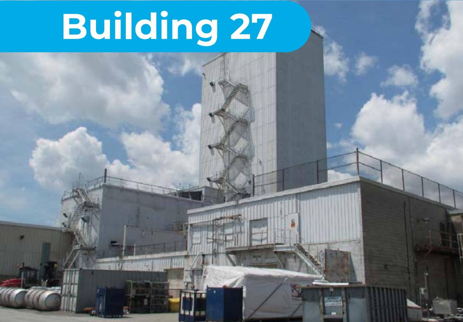
This is **Building 27**, Cameco's out of service  $UF_6$  plant. Work on this building so far has been focused on asbestos removal and removal of equipment.
