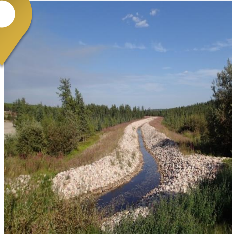
McArthur River – Treated water flow path. (Photo source: CNSC)
