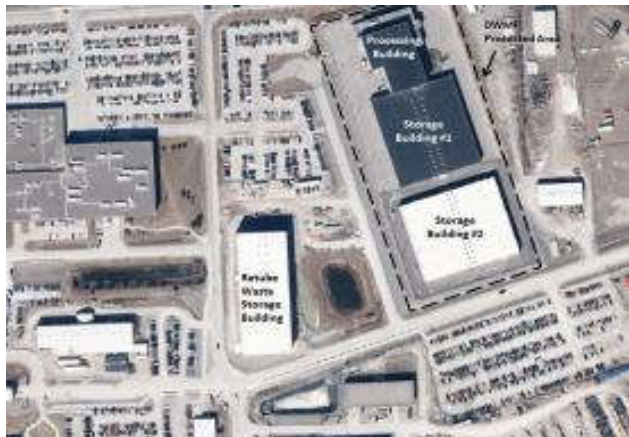
Darlington Waste Management Facility (DWMF)
