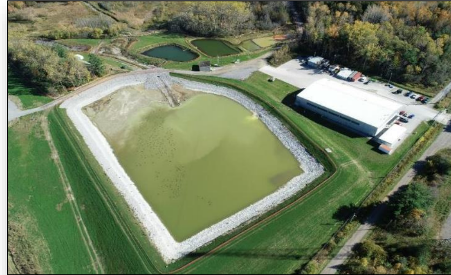
Waste Water Treatment Plant
