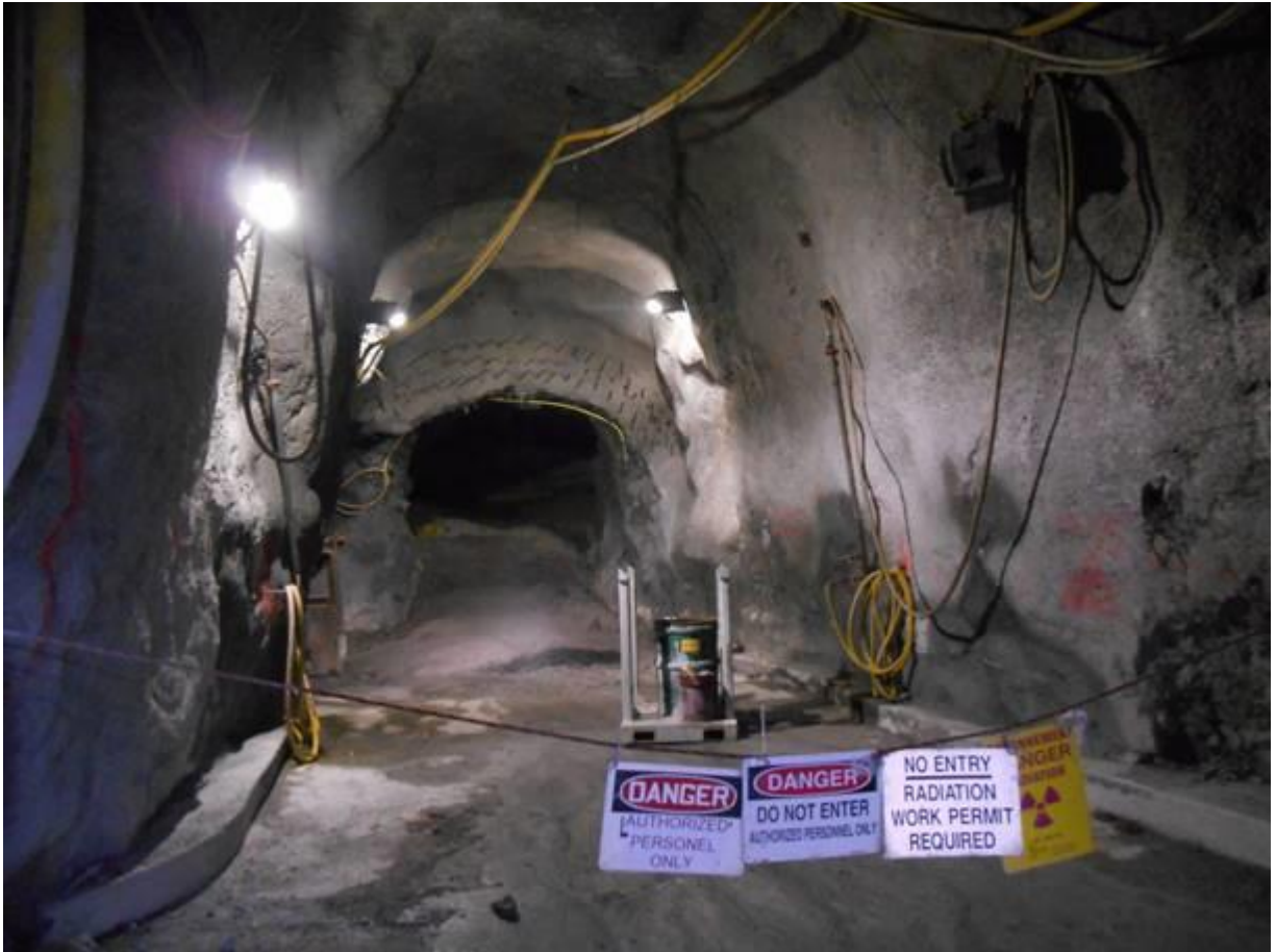
Figure 2.13: Warning signage in underground work area
