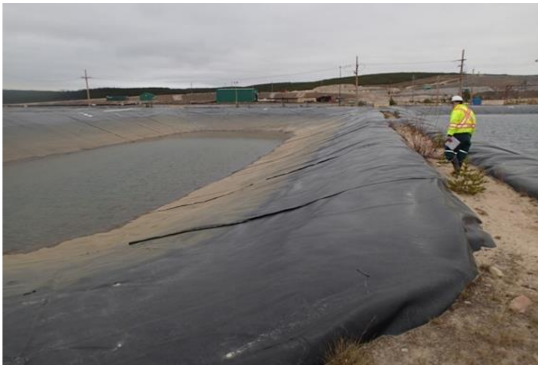
Figure 4.3: McArthur River Operation - monitoring pond
