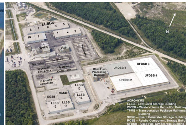
Western Waste Management Facility (on Bruce site) (WWMF)
