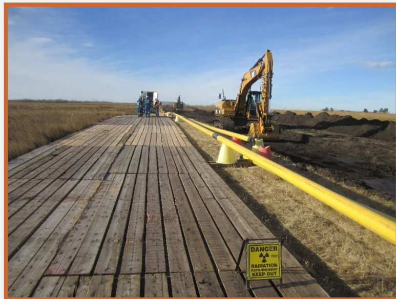
A licensee setting up for industrial radiography operations ( source: CNSC staff )
