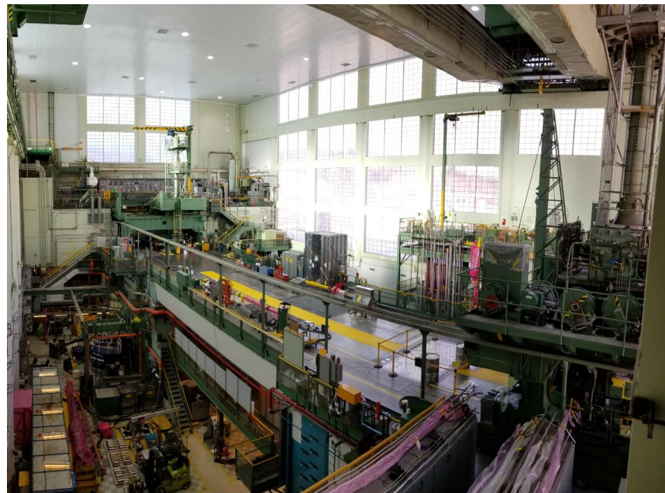
The NRU reactor hall
