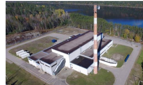
Nuclear Power Demonstration, Rolphton, Ontario
