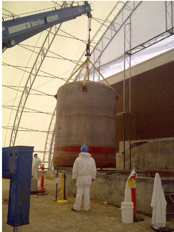
Figure 2-3 : ALWTC Tank TK-816 Removal.
