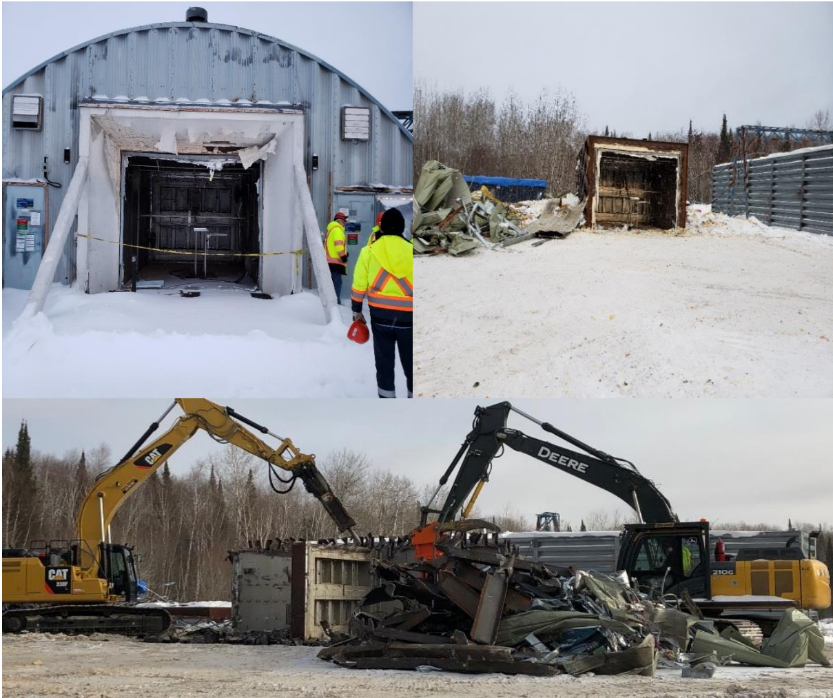
Figure 2-12 : Decommissioning LSVCTF facilities (winter 2018/19)
