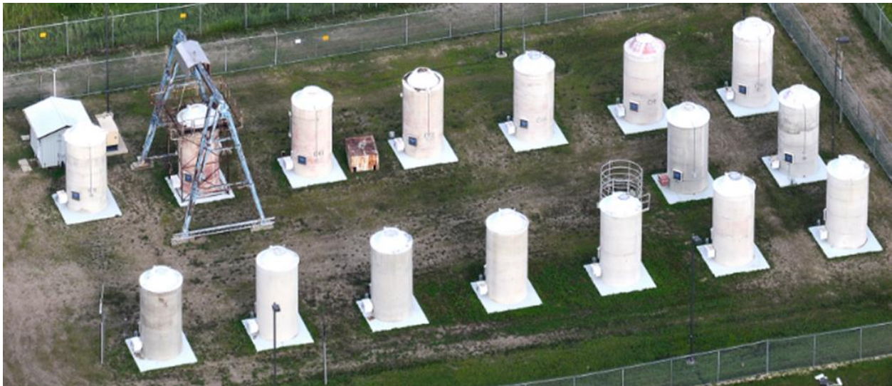
Figure 3-1 : Concrete Canister Storage Facility
