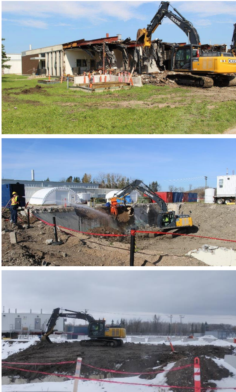
Figure 2-7 : Laundry & Decontamination Building Demolition (2017)
