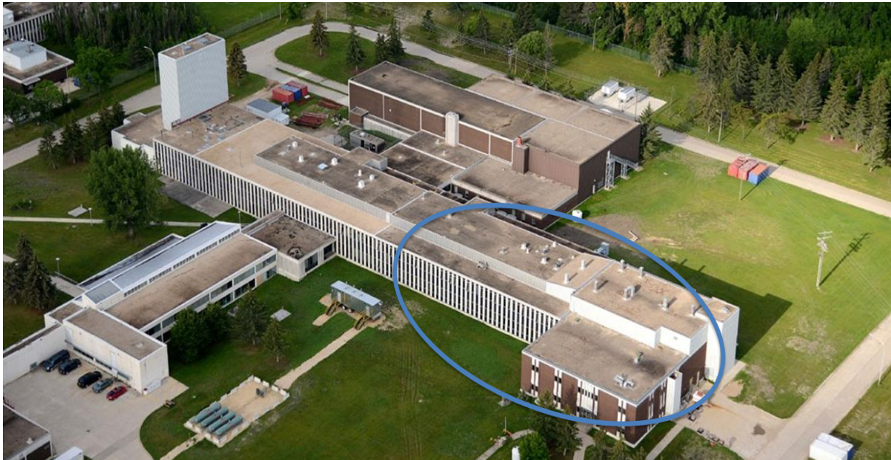
Figure 2-8 : Building 300 Stages 4 and 7 Prior to Demolition
