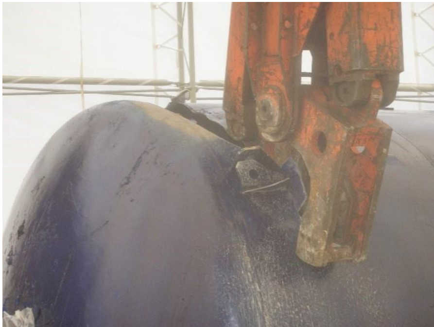
Figure 2-4 : Size-Reduction of TK-816 for Storage
