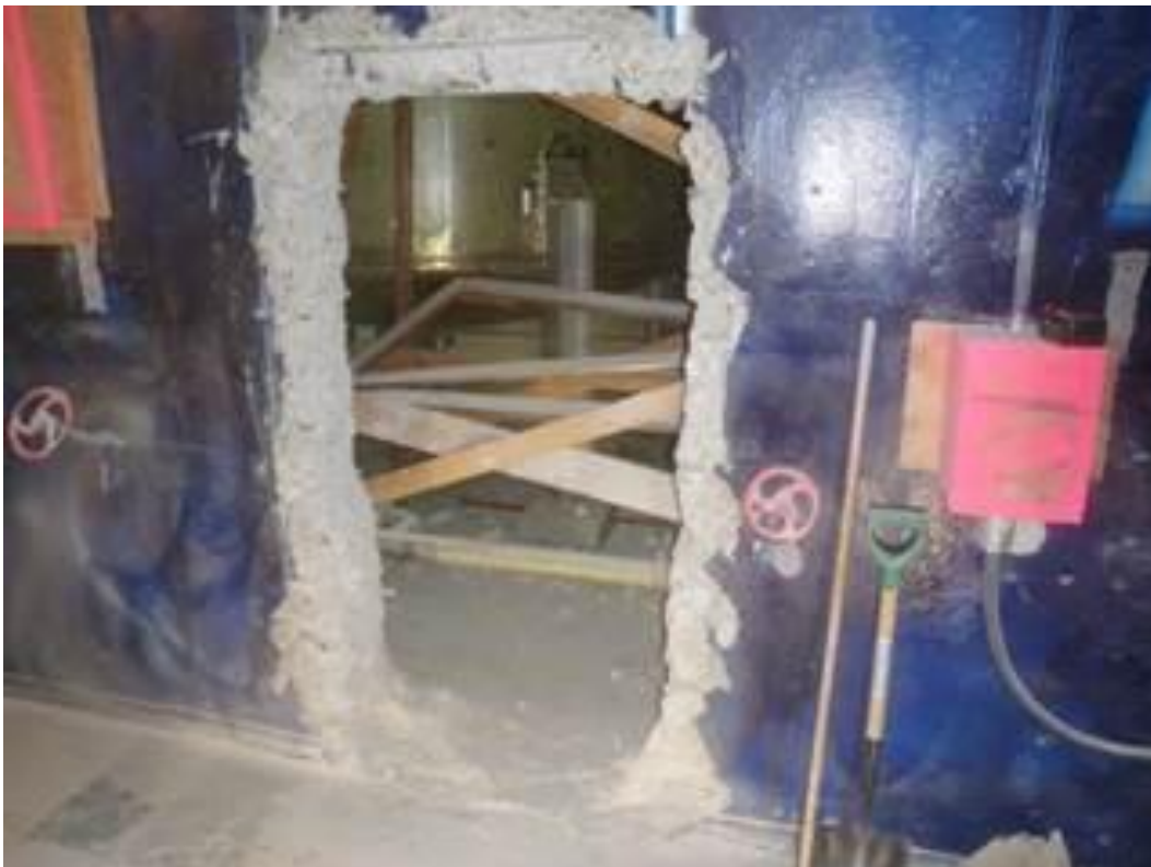
Figure 2-6 : Additional access doorway into ILLW process cell
