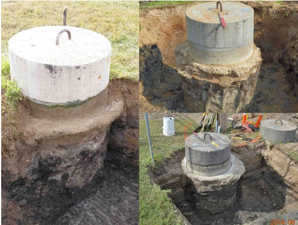
Figure 3-10 : WMA Standpipes – Pre-Decommissioning Condition Assessment
