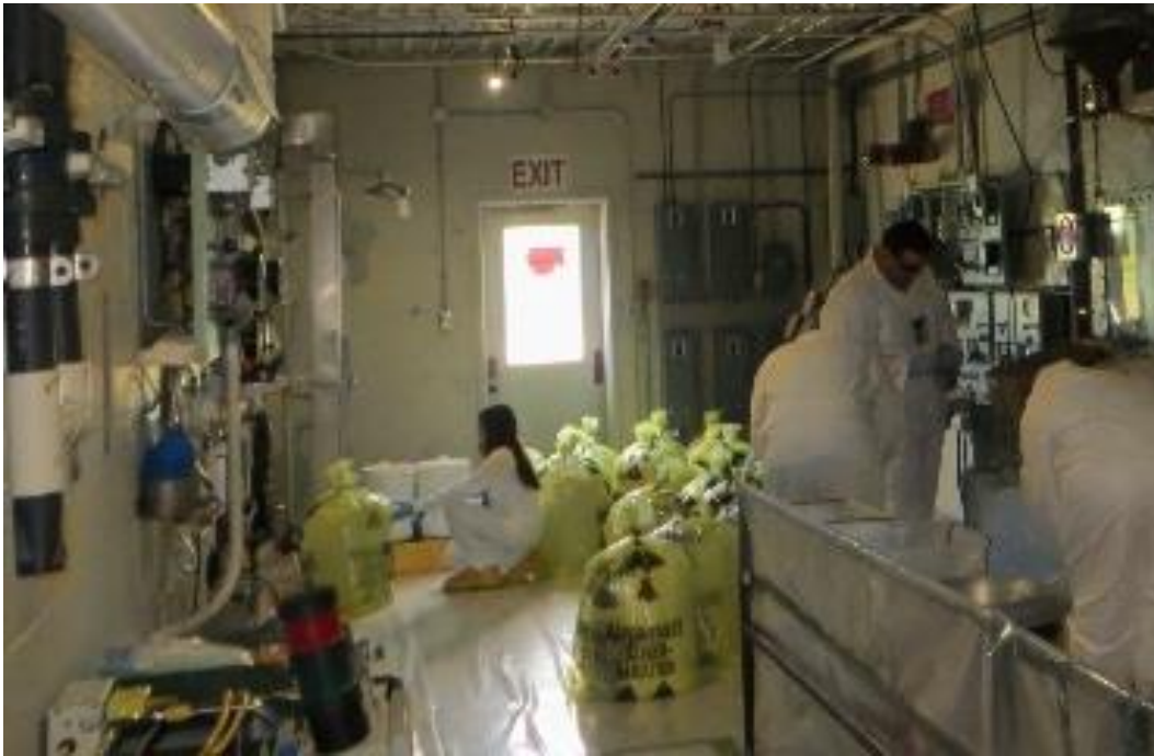
Figure 2-5 : Decommissioning the interior of the ALWTC upper operations gallery
