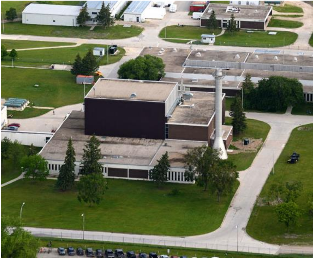
Figure 3-22 : WR-1 Building (B100) [viewed from the south]
