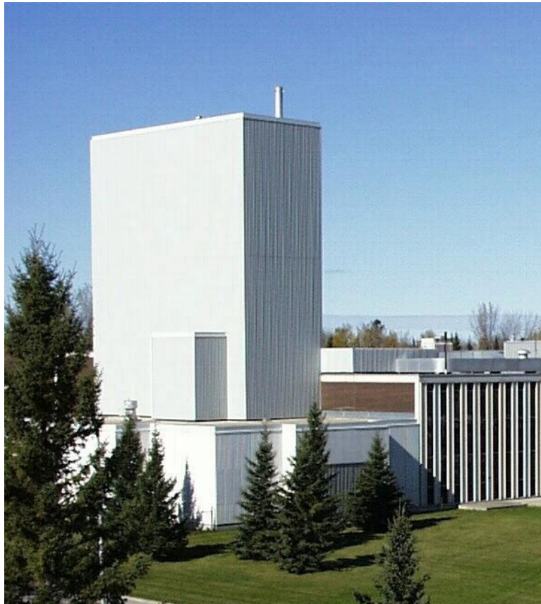
Figure 2-11 : RD-14M Thermalhydraulics Laboratory – South End of Building 300
