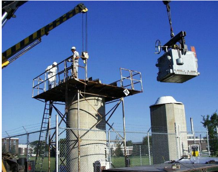
Figure 3-3 : Mock trial of fuel basket retrieval from canister in 2017
