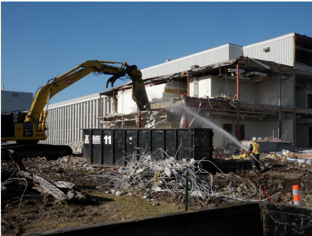
Figure 2-10 : Building 300, Stage 7 Demolition in Progress (Water Used for Dust Suppression)
