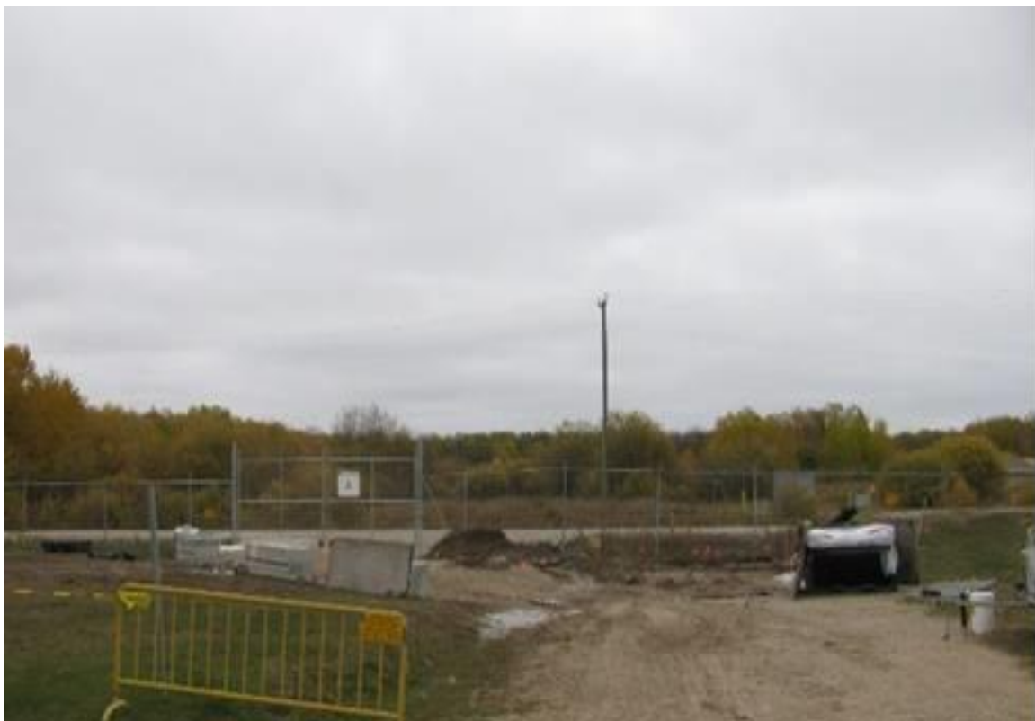
Figure 2-13: Organic Incinerator, Before and After Decommissioning
