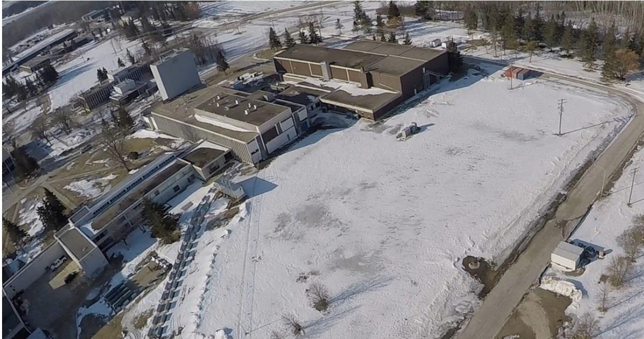
Figure 2-9 : Building 300 After Demolition of Stages 4 and 7
