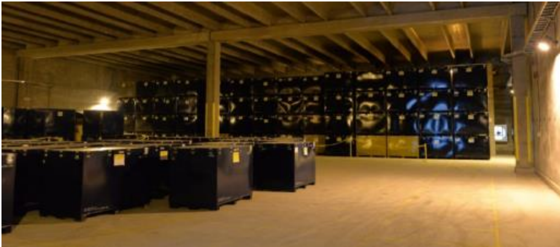
Figure 3-7 : Waste Containers in SMAGS (WMA Building 923)
