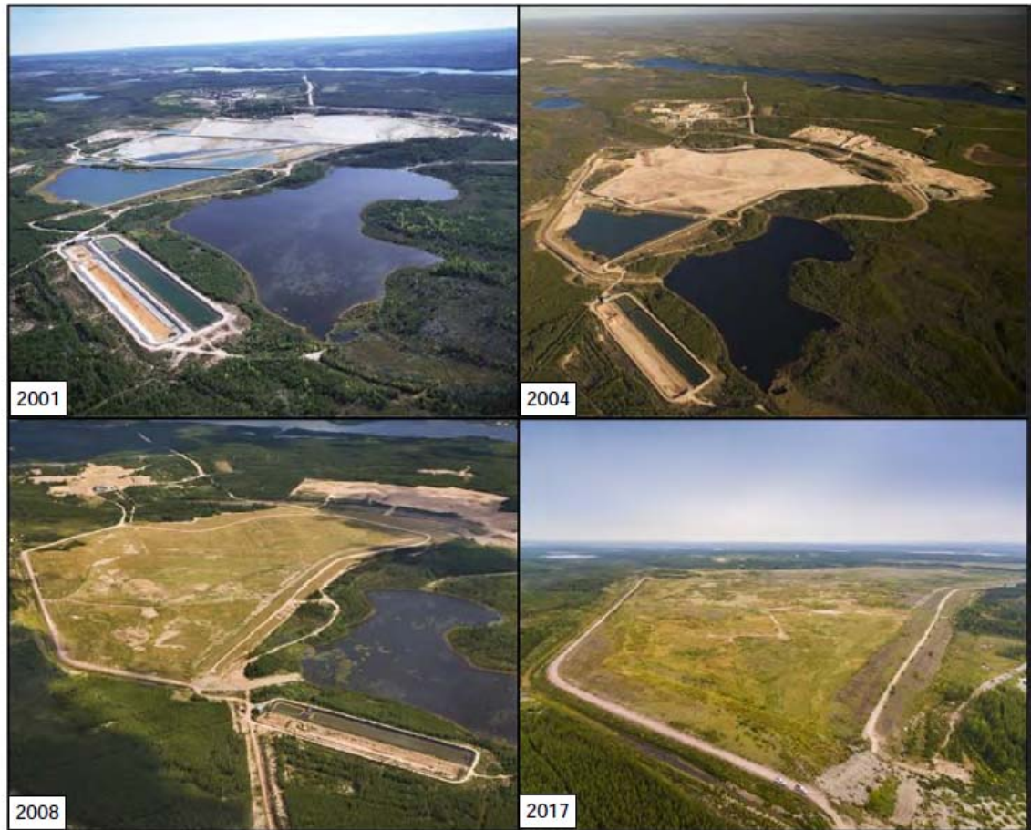
Figure 2 - Cluff Lake Project - Aerial photographs of tailings management area (source: Orano Canada Inc.)
