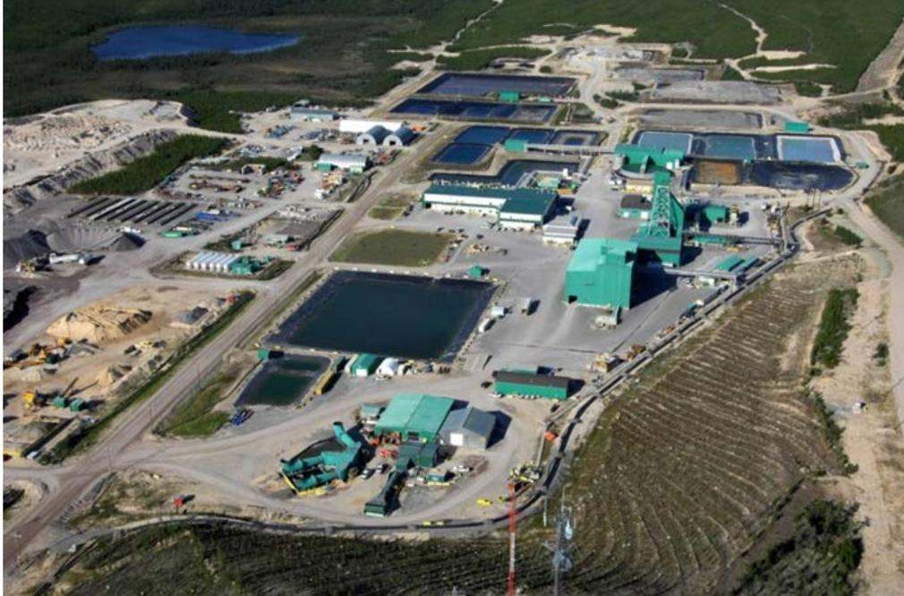
High-grade uranium ore is mined, mixed with water and ground in a ball mill to form slurry, and pumped to the surface. The ore slurry is loaded into containers and transported to the Key Lake Operation for further processing.
