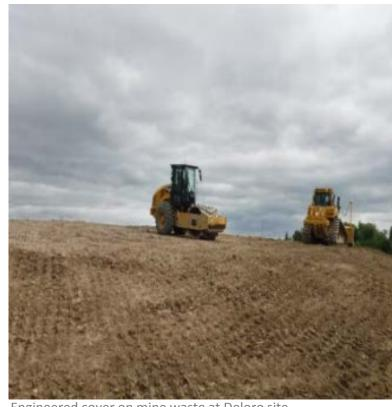
Engineered cover on mine waste at Deloro site. (Photo source: CNSC)
