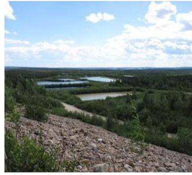
Polishing ponds at the Rabbit Lake Operation as seen from the above ground tailings facility berm. (Photo source: CNSC)
