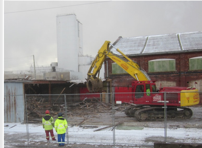
Demolition of building 42 on the Centre Pier in Port Hope.
