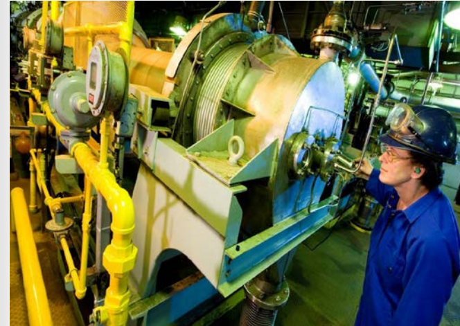
Port Hope Conversion Facility worker performing visual check on \text{UO}_2 inside rotary kiln.
