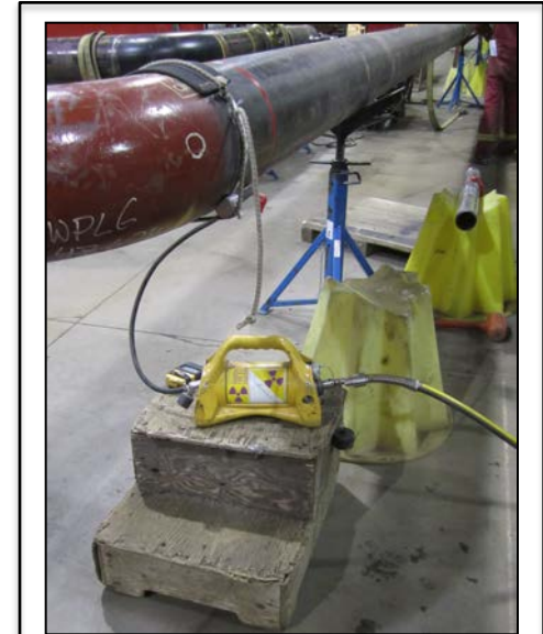
Exposure device being used for non-destructive testing (Source: CNSC)
