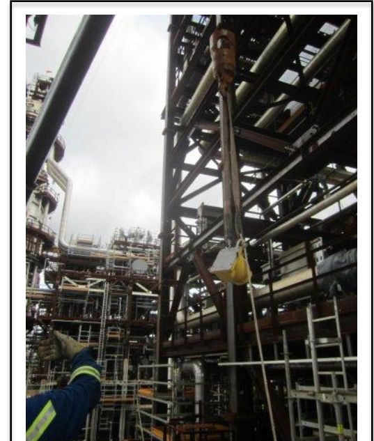
Installation of a fixed gauge by a servicing company (Source: CNSC)
