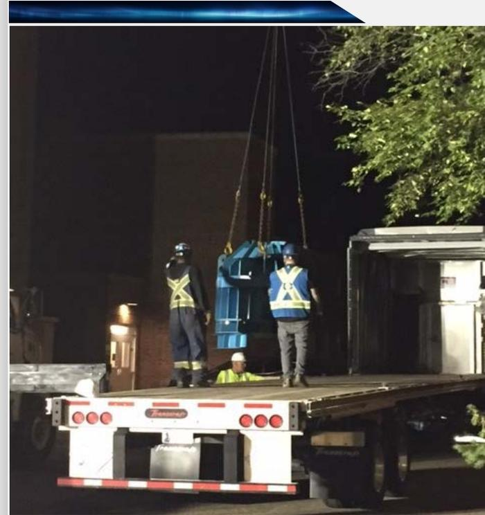
Loading of the shielded reactor core in preparation for shipping it to the United States.
