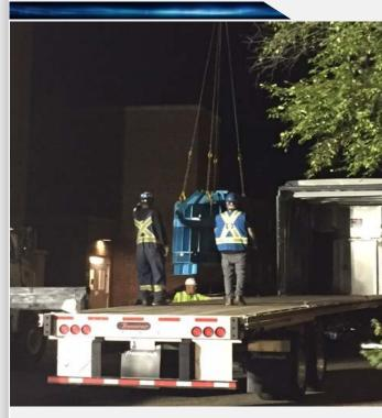
Loading of the shielded reactor core in preparation for shipping it to the United States. Photo: University of Alberta
