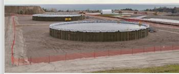
Two of six temporary 6,000 m<sup>3</sup> tanks. (Photo courtesy CNL)
