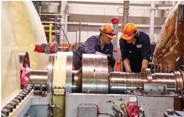
Figure 14 - Turbine maintenance
