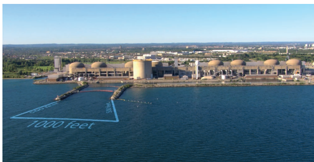
Figure 17 - Fish Diversion System
