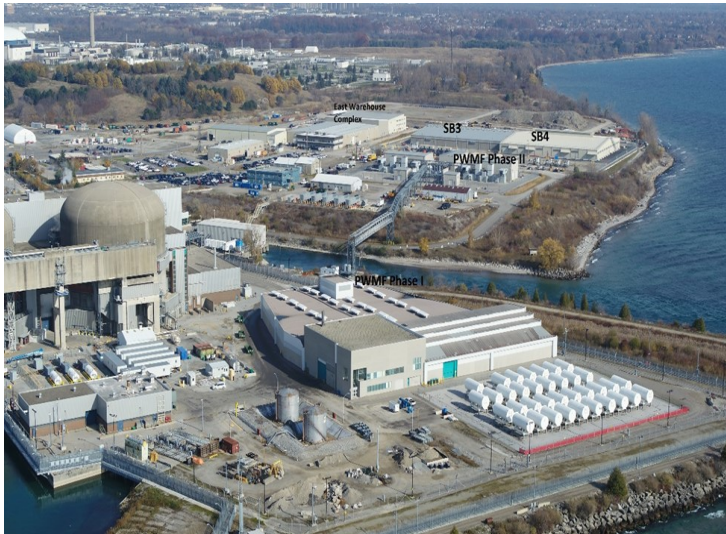
Figure 6: Pickering Waste Management Facility
