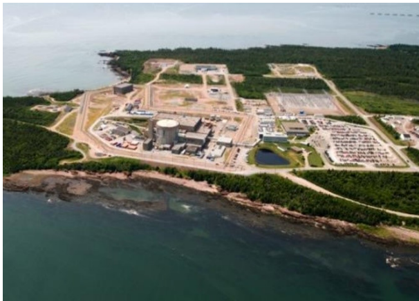
Figure 9: Point Lepreau Nuclear Generating Station
