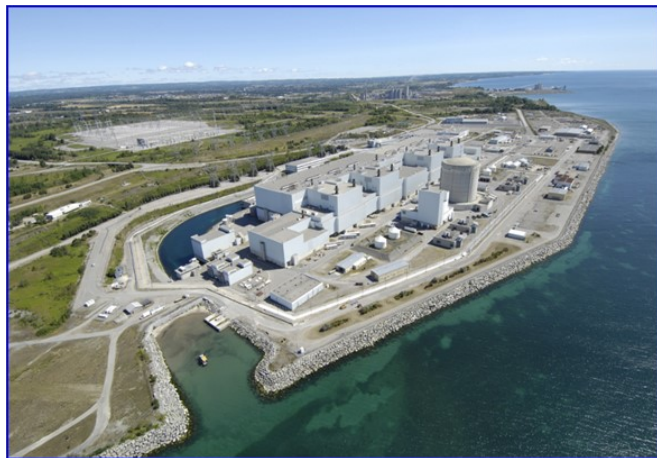
Figure 4: Darlington Nuclear Generating Stations
