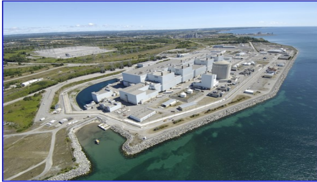
Figure 3: Darlington Nuclear Generating Stations
