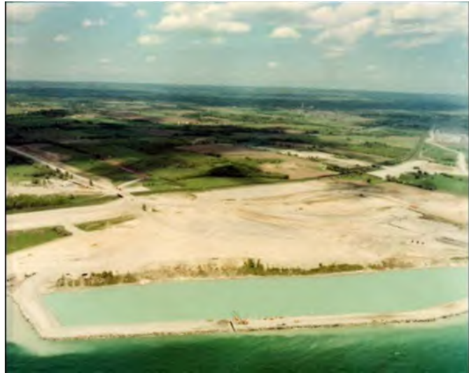
Cofferdam Construction for DNGS
