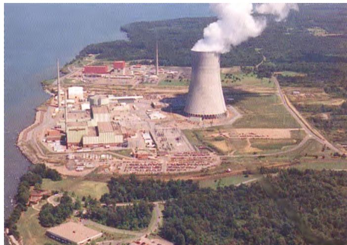
Natural Draft Cooling Tower at Nine Mile Point, NY (Nuclear Tourist Web Site 2008)
