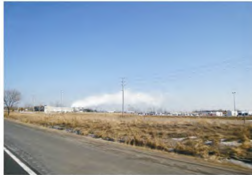
Natural Draft Cooling Towers Highway 401 Eastbound, Facing South-East (No-Foliage)
