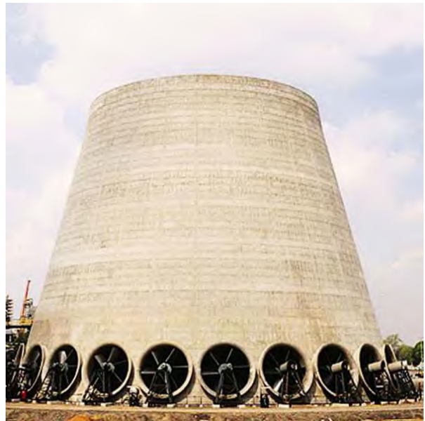
Fan Assisted Natural Draft Cooling Tower (SPX Cooling Technologies 2008)
