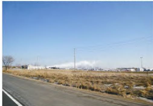
Mechanical Draft Cooling Towers Highway 401 Eastbound, Facing South-East (No-Foliage)
