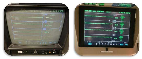
Figure 40: Old CRT display (left) and new touchscreen display (right)
