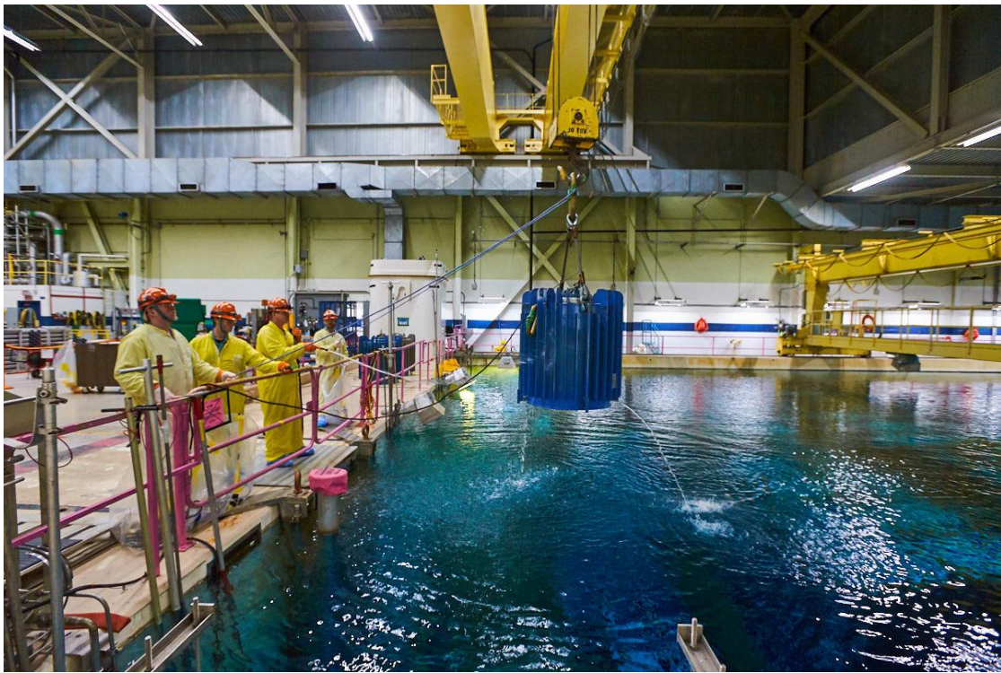
Co-60 Lifted from the IFB at Pickering NGS
