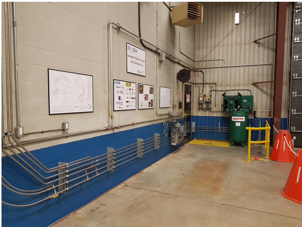
Figures 5&6: These images depict and demonstrate the IPS mock-up which is assembled to validate working principles of the system. After detailed design is completed, changes will be made to the mock-up to accurately represent the system that will be installed at Bruce Power. This Isogen Facility will provide hands on training for the required personnel.
