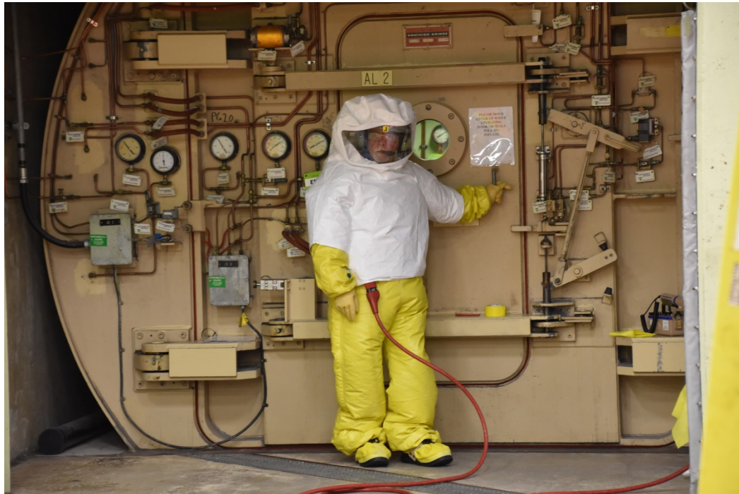
Figure 10: Employee Equipped with Personal Protective Equipment Entering the Vault
