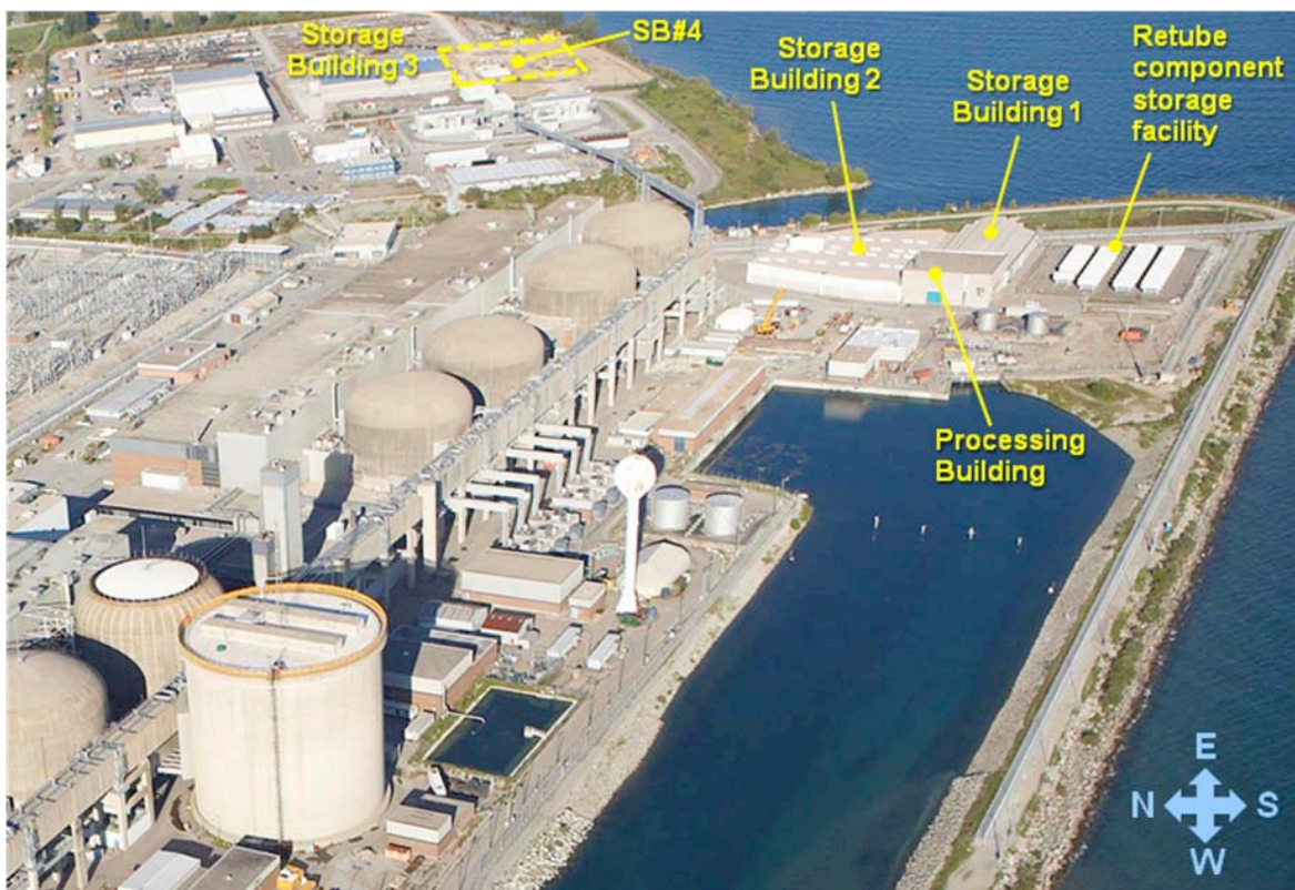
Figure 4.5 – PWMF I (Processing Building, Storage Buildings 1 and 2 and Retube Component Storage Facility) and PWMF II (Storage Building 3 and future Storage Building 4) area
