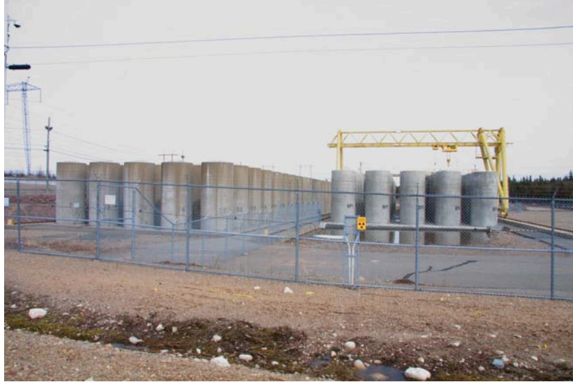
Figure 4.8 – Point Lepreau spent fuel dry storage area
