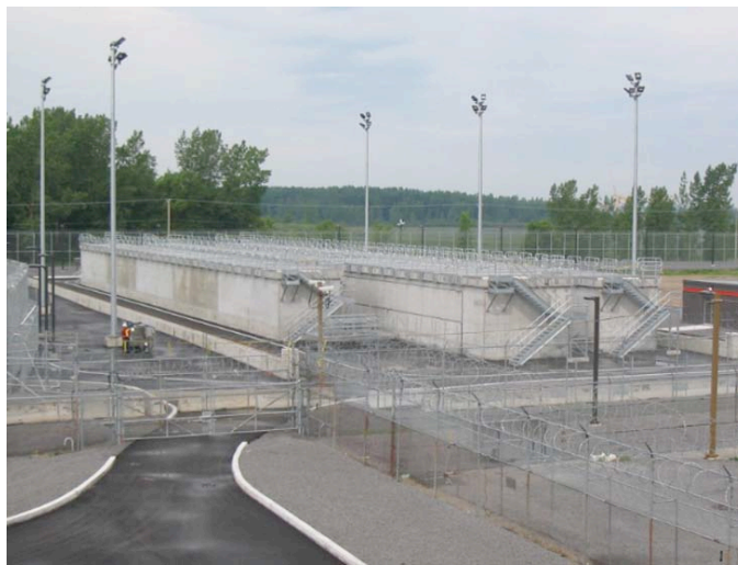
Figure 5.3 – Gentilly-2 spent fuel dry storage area and low-level radioactive WMA
