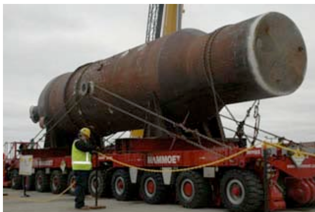
Figure H.2 – Steam generator being transported near the plant as part of the refurbishment
