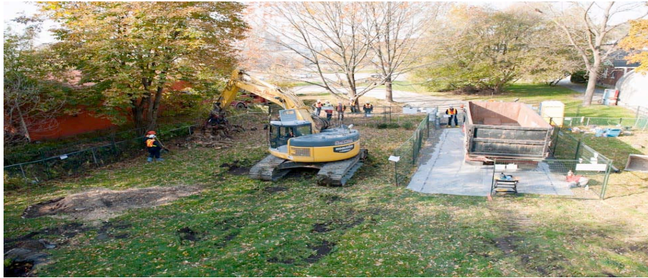
Figure K.5 – Port Hope trial remediation
