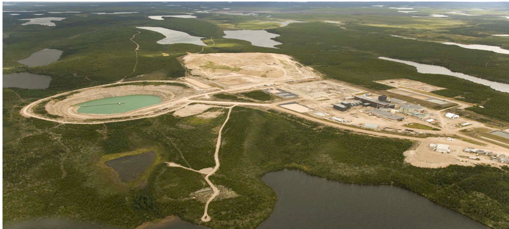
Figure 6.3 (a) – JEB Tailings Management Facility at McClean Lake
