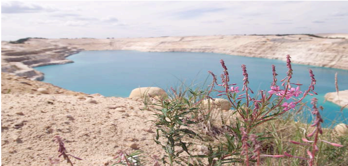
Figure 6.1 – Deilmann Tailings Management Facility at Key Lake
