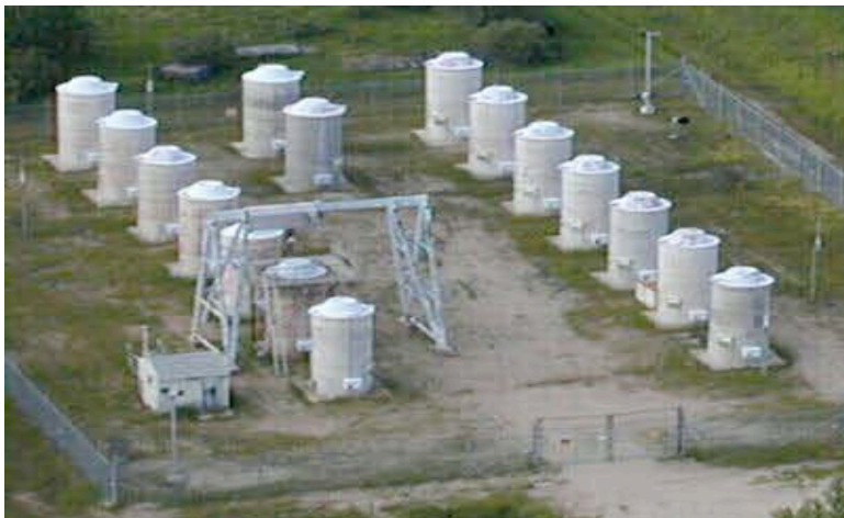
Figure 4.10 – Whiteshell Laboratories Concrete Canister Storage Facility (CCSF)
