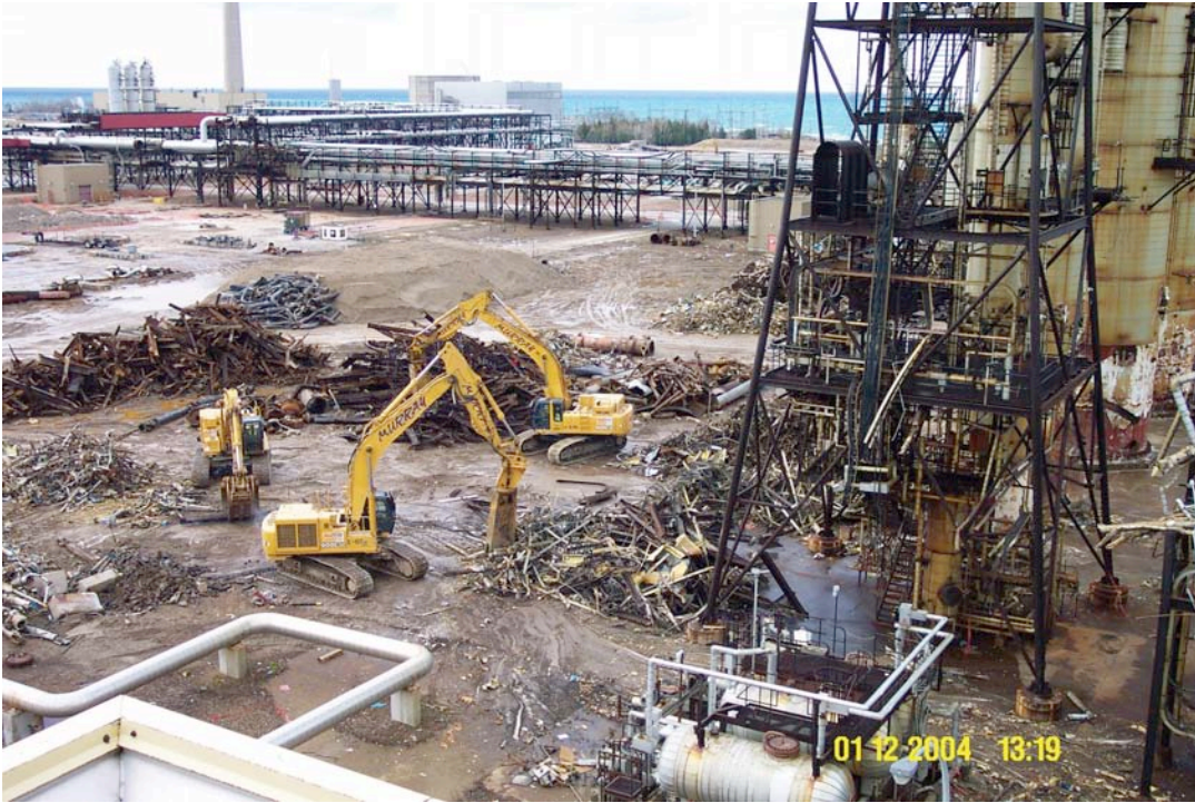
Figure 7.5 – Demolition of the Bruce Heavy Water Plant site
