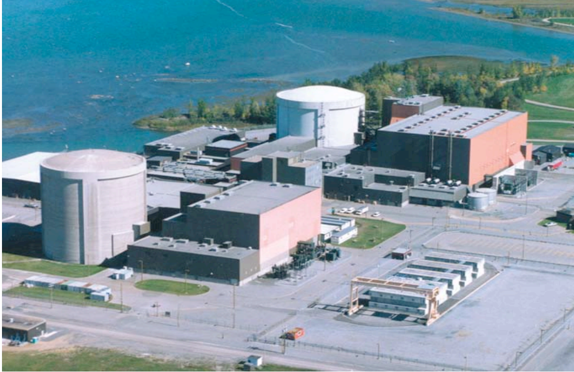
Figure 4.7 – Gentilly-2 spent fuel dry storage facility (bottom right)
