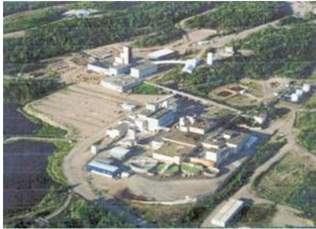
Figure 8.6 (a) – Aerial view of the Stanleigh Mine site prior to decommissioning
