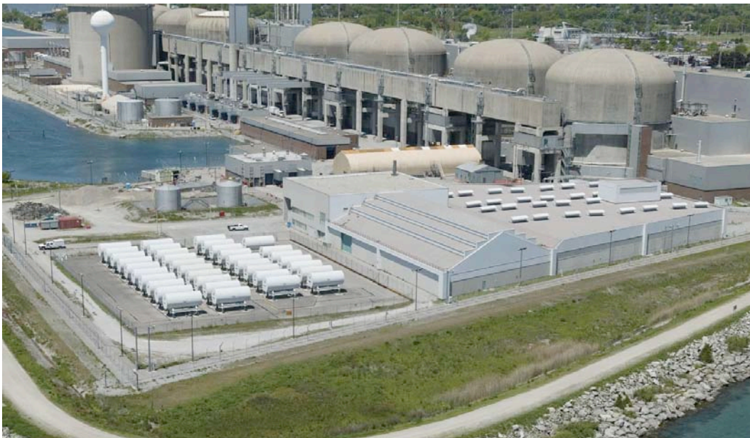
Figure 5.1 – Pickering Waste Management Facility, with RCSA (left) and spent fuel dry storage area (right)
