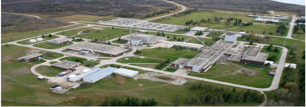
Figure 7.1 – Aerial view of Whiteshell Laboratories main site
