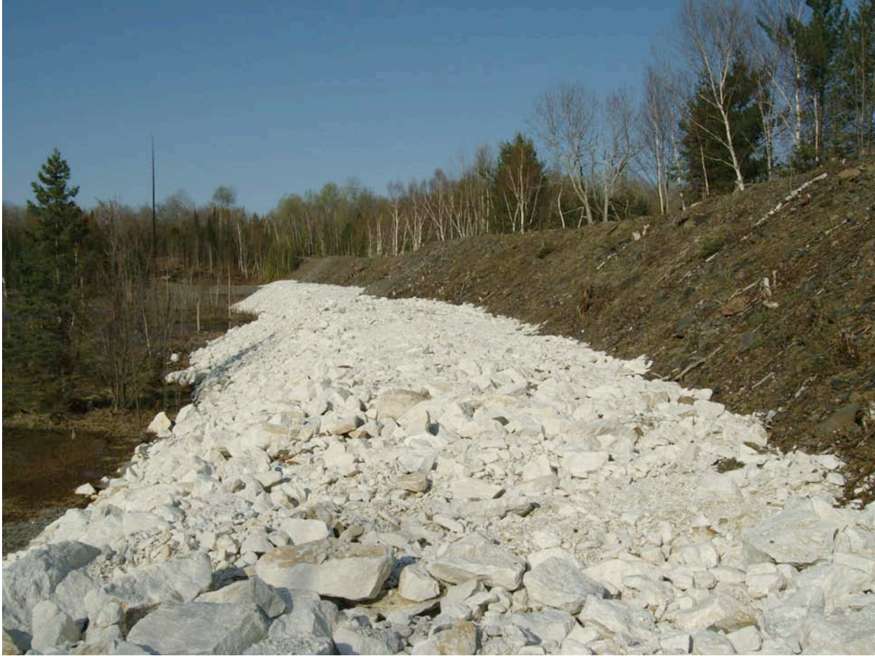
Figure 8.7 – Main tailings dam Dyno Mine site
