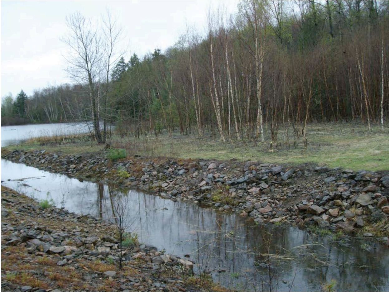
Figure 8.8 – South Tailings Basin Spillway at Bicroft Tailings Storage Facility
