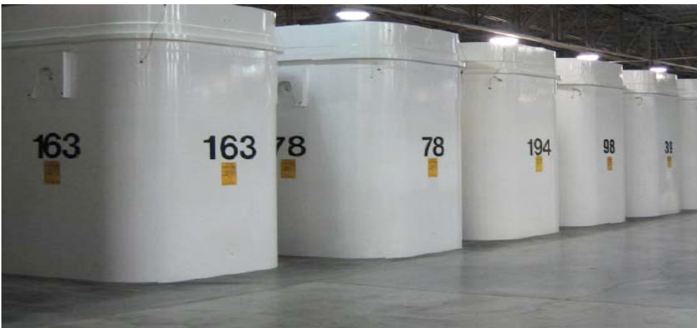
Figure 4.4 – Dry storage containers at the Pickering Waste Management Facility
