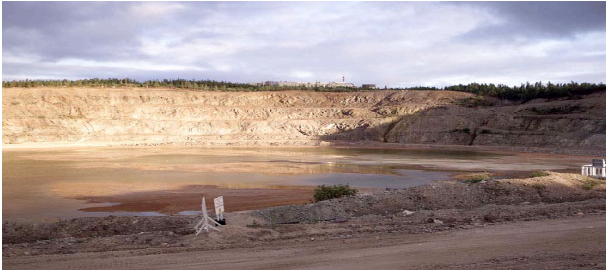
Figure 6.2 (a) – Rabbit Lake In-pit Tailings Management Facility
