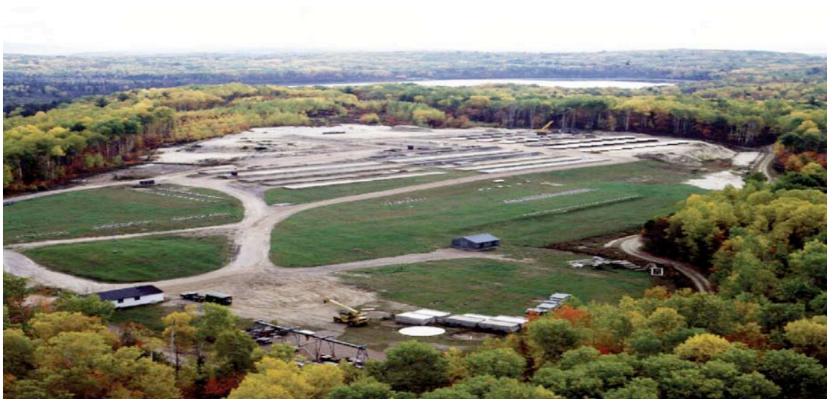
Figure 5.6 – Waste Management Area B at the CRL site
