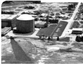
Early prototype reactors (NPD, Douglas Point)
