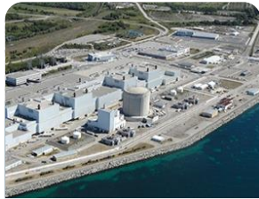
Commercial power reactors (Pickering, Darlington, Bruce, Point Lepreau, Gentilly-2)
