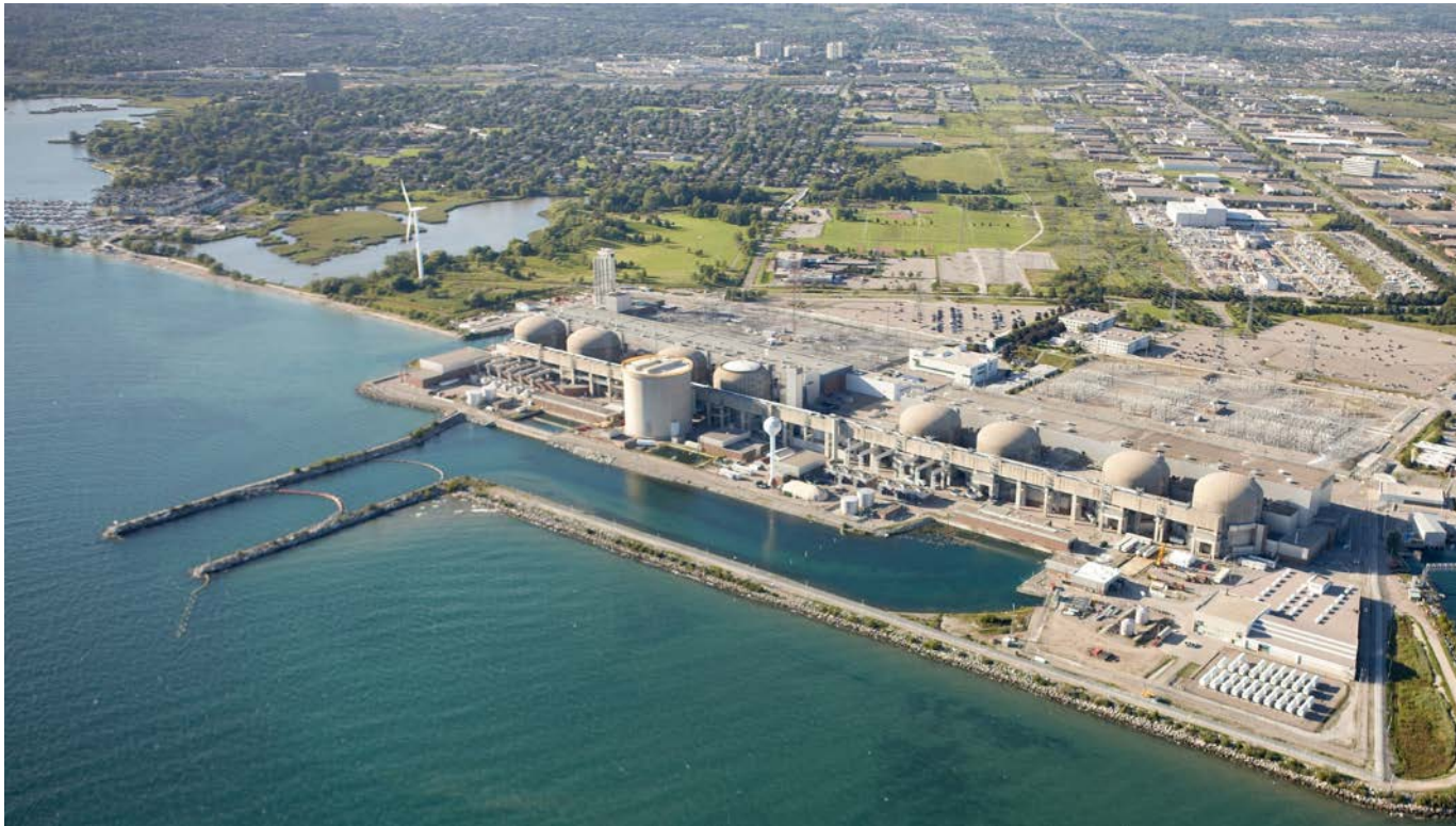
Pickering Nuclear Generating Station
