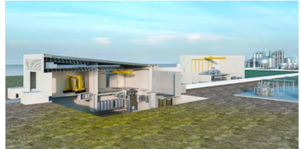
Example of an SMR technology: Facility cross-section Terrestrial Energy Integral Molten Salt Reactor (IMSR-4000) – (Courtesy of Terrestrial Energy)
