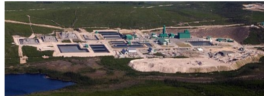
Above: Key Lake Mill, below: McArthur River Mine
