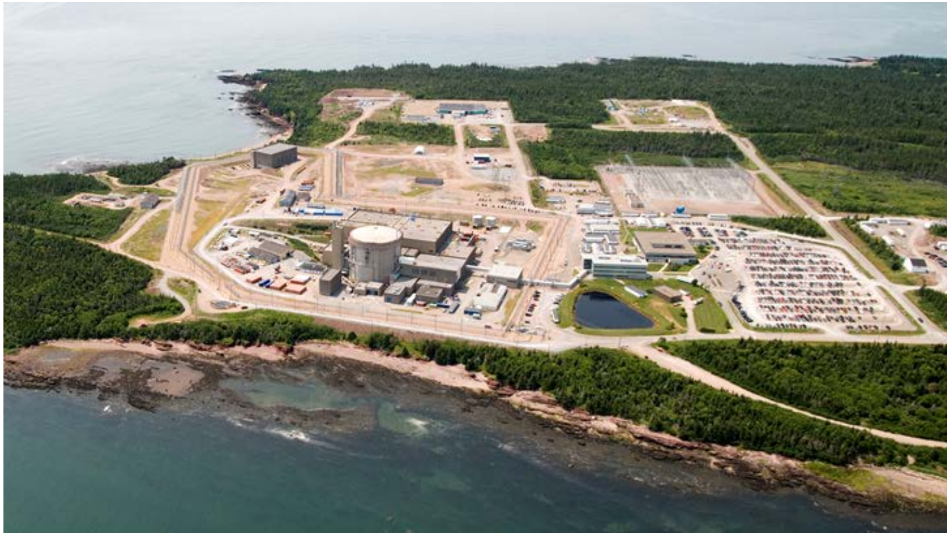
Point Lepreau Nuclear Generating Station
