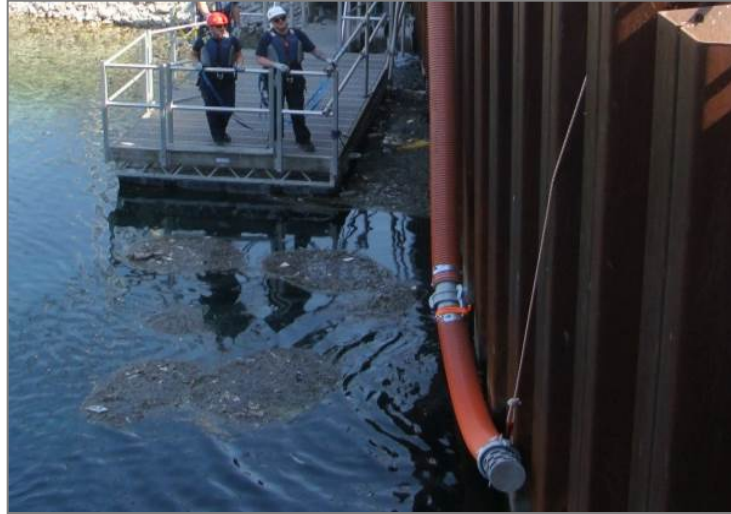
Darlington emergency water supply
