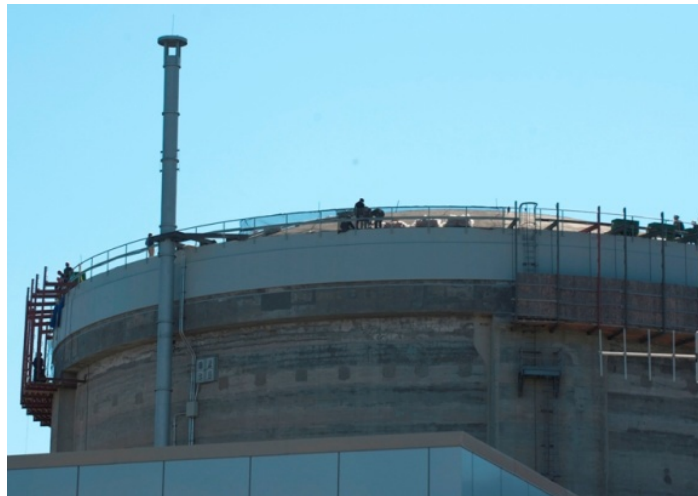
Point Lepreau Emergency filtered vent stack
