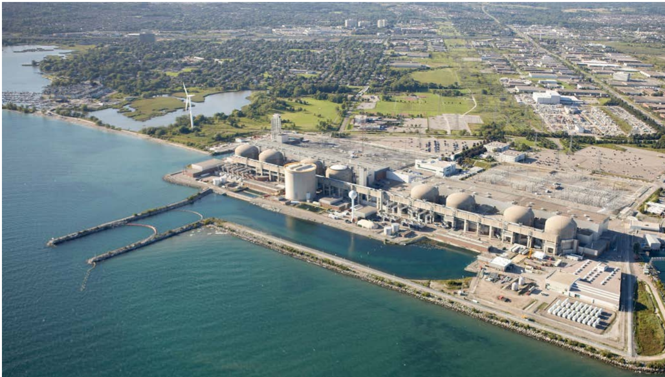
Aerial view of Pickering Nuclear Generating Station
