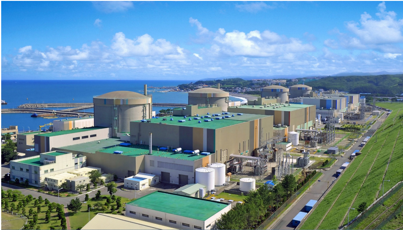
Wolsong Nuclear Power Plant, Republic of Korea
