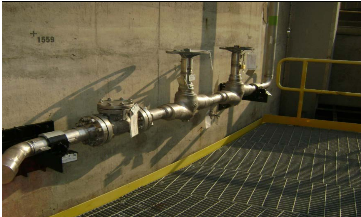
Point Lepreau calandria vault make-up
