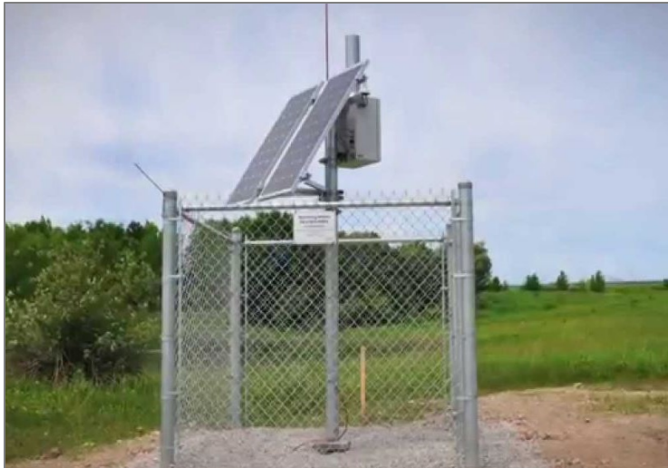
Real-time radiation monitoring
