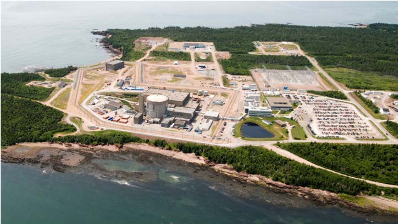
Aerial view of Point Lepreau Nuclear Generating Station
