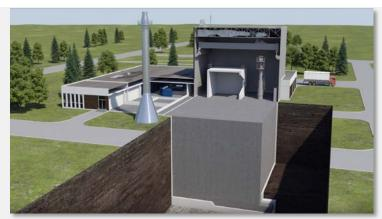
Because it is primarily located low grade the majority of contamination is in the reactor core the entire below grade portion will be filled with grout.
