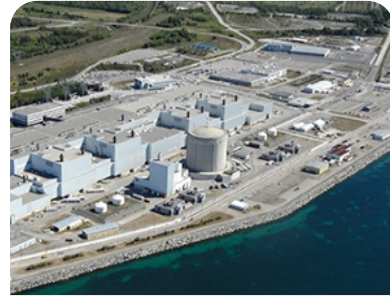
Commercial power reactors (Pickering, Darlington, Bruce, Point Lepreau, Gentilly-2)
