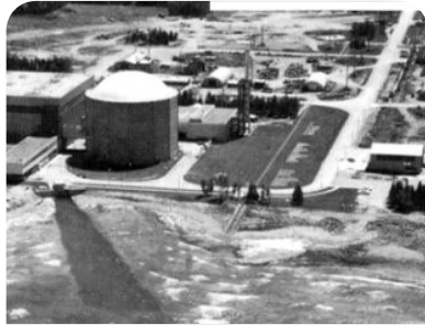
Early prototype reactors (NPD, Douglas Point)
