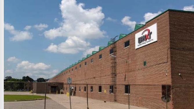
BWXT buildings in Toronto (top) and Peterborough (bottom).
