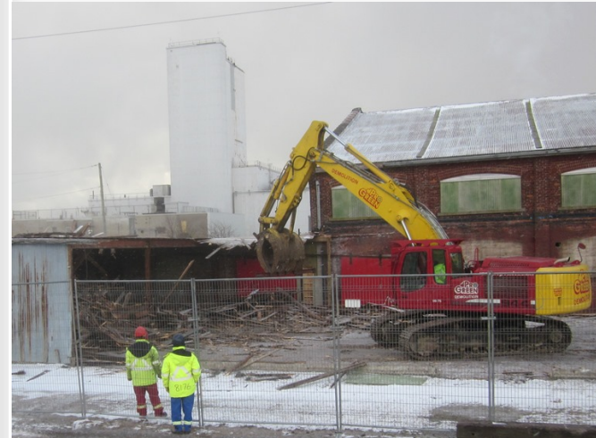
Demolition of building 42 on the Centre Pier. Photo source: Cameco
