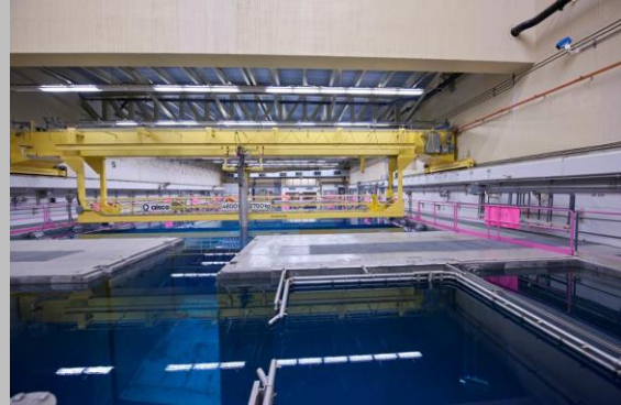
A typical Canadian irradiated fuel bay.
